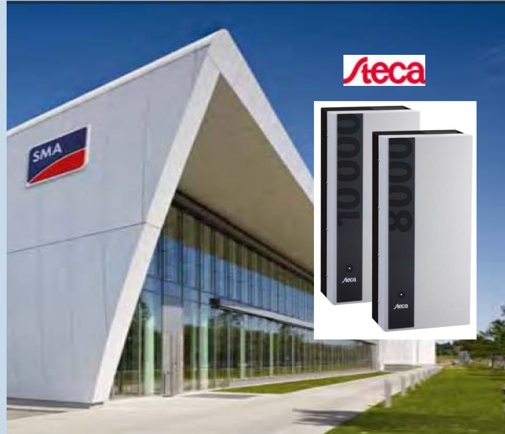
Fig. 1 - The new 4 GW inverter factory of SMA Solar technology AG was officially opened in July 2009; the plant is designed to work CO 2 -free and is therefore equipped with a 1.1 MW PV system and a biogas CHP unit (photo: SMA Solar Technology AG).
