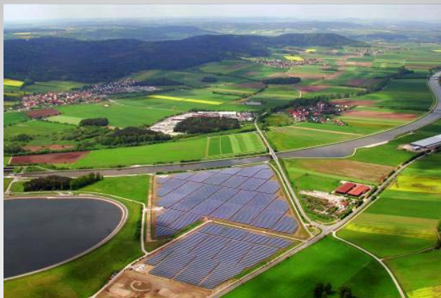
Muehlhausen, Bavaria, Germany, 6 MW SunPower T0 Tracker
