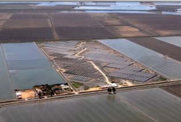
Isla Mayor Spain, 8.4 MW SunPower T0 Tracker
